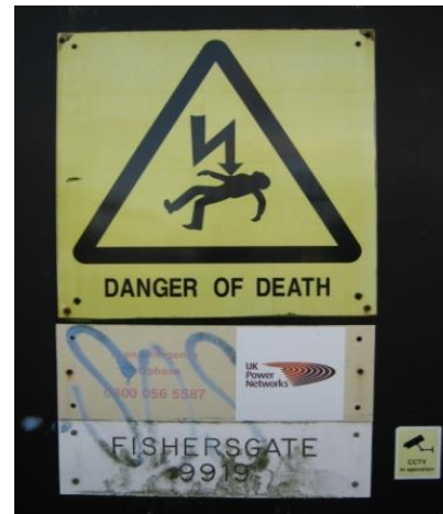
Figure 2 - Vandalised Sign with graffiti
