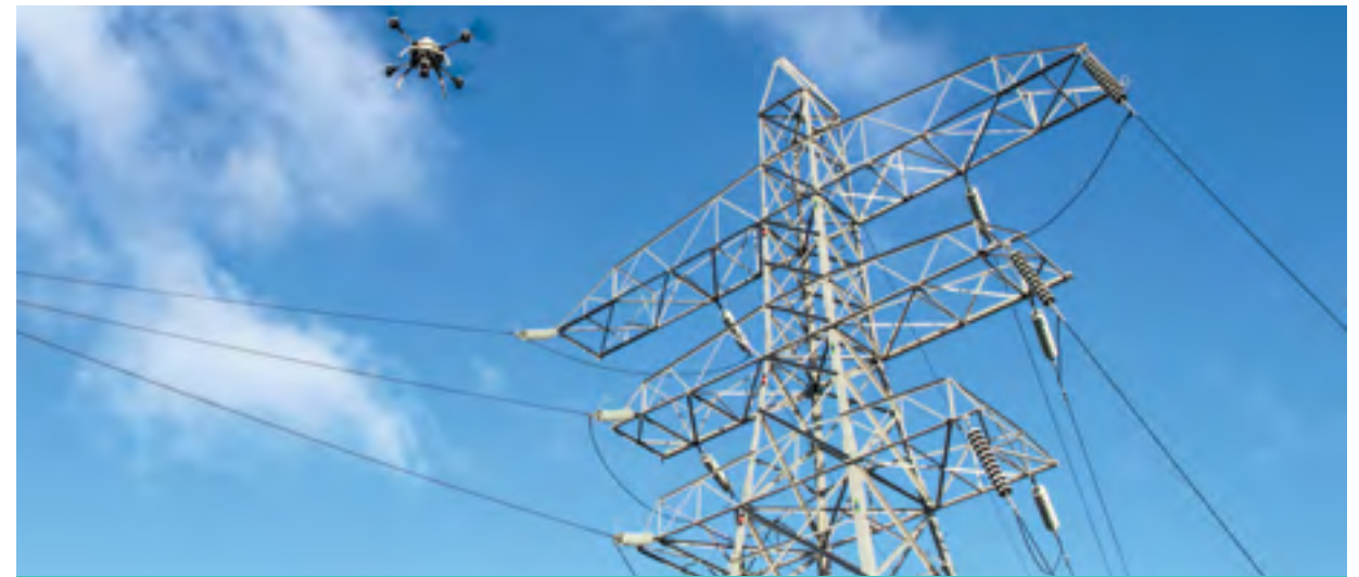
Improvements to efficiency by using small remote controlled helicopters to carry out overhead line inspections.
