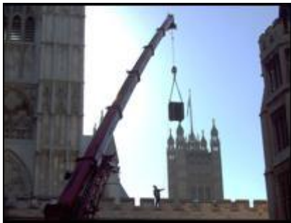
Figure 25: Plant moving over the top of Westminster Abbey by crane
