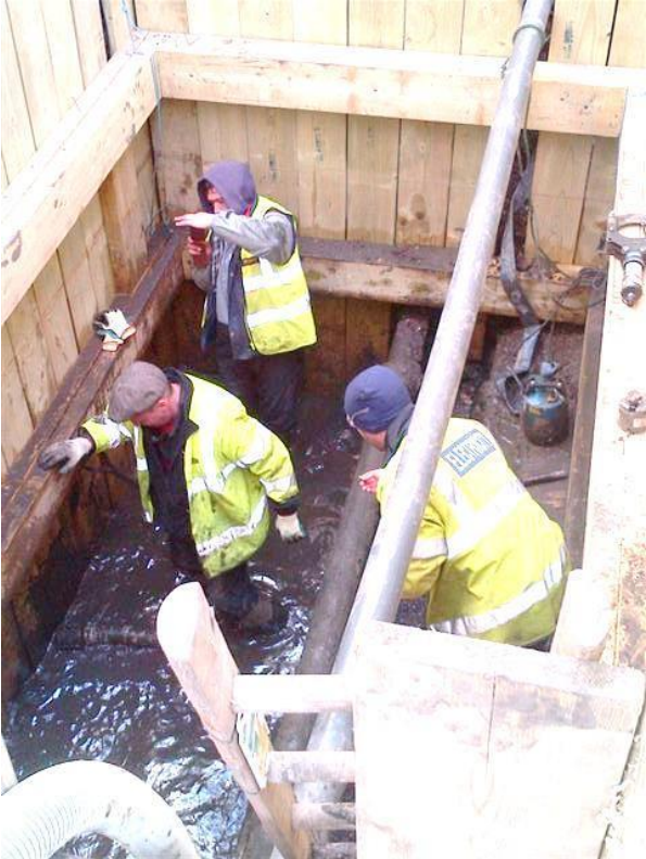
Figure 20: The extreme conditions of one of the HV joint holes
