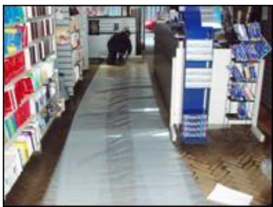
Figure 26: Preparation of plant access through a bookshop in Great Marlborough St SW1
