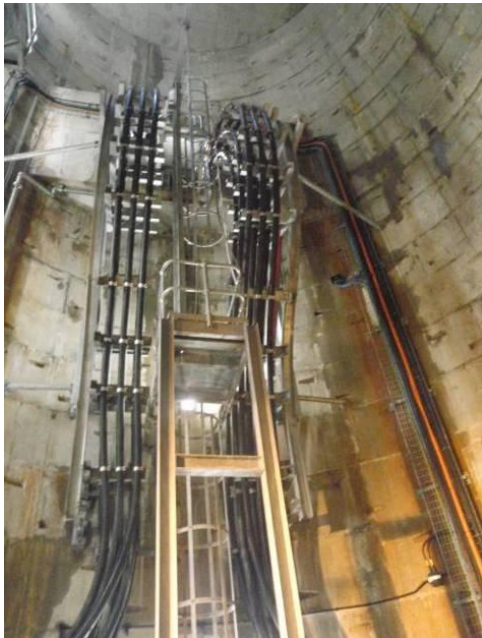
Figure 52: Tunnel, Shaft Olympic Park
