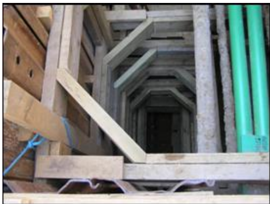
Figure 35: EHV cable fault repairs Backhill to Fisher St
