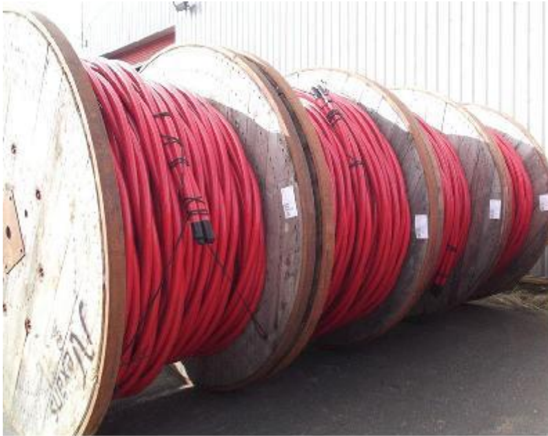
Figure 18: Drums of HV Triplex Cable
