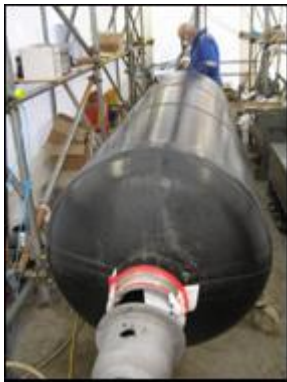
Figure 31: Oil transition joint being prepared at Dartford cable fire
