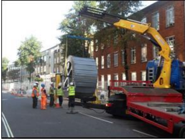
Figure 38: Road closure required for delivery of replacement cable
