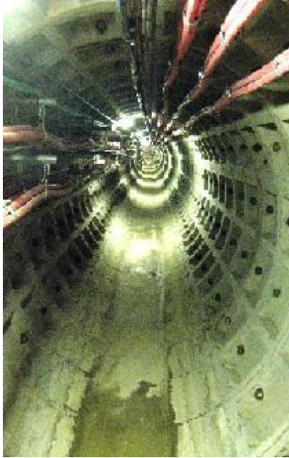
Figure 53: Millennium Cable Tunnel Inspection
