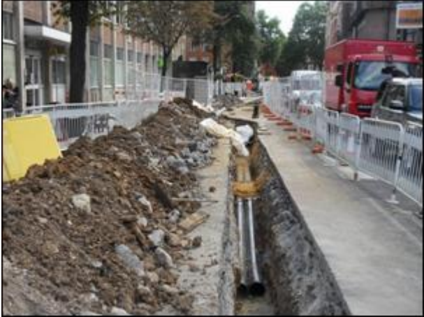
Figure 37: Road Excavation Lisson Grove
