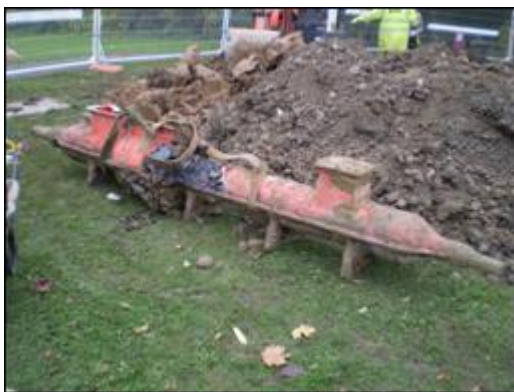
Figure 39: Original Gas joint failure
