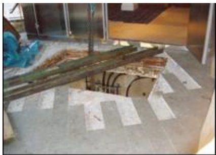
Figure 27: Royal Lancaster Hotel plant replacement
