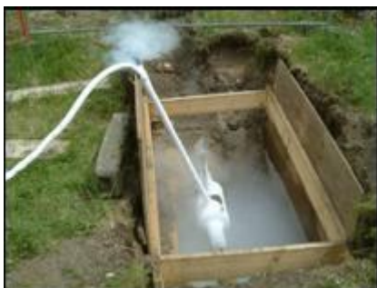
Figure 32: A Cable freeze in progress on a shallow cable route
