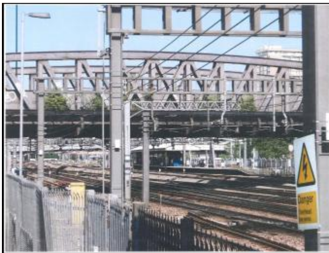
Figure 43: Ranelagh Railway Bridge
