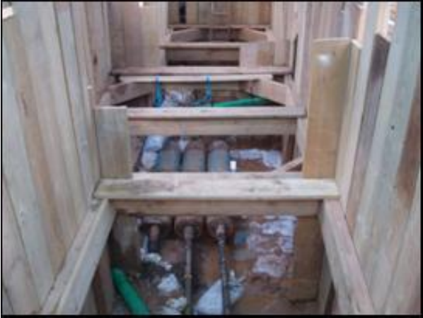
Figure 41: New Cable route circa 2m deep
