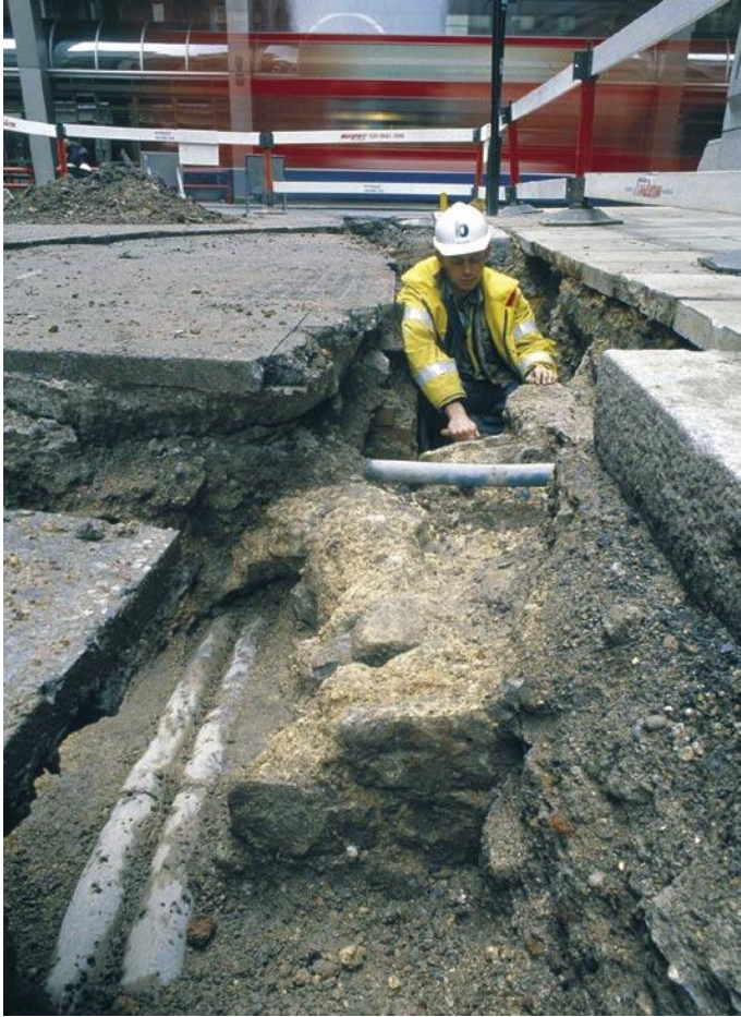
Figure 7: City wall, Goring Street
