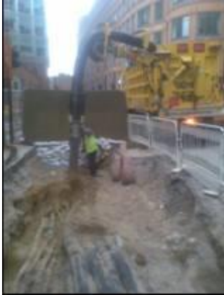
Figure 22: Vacuum excavator being used
