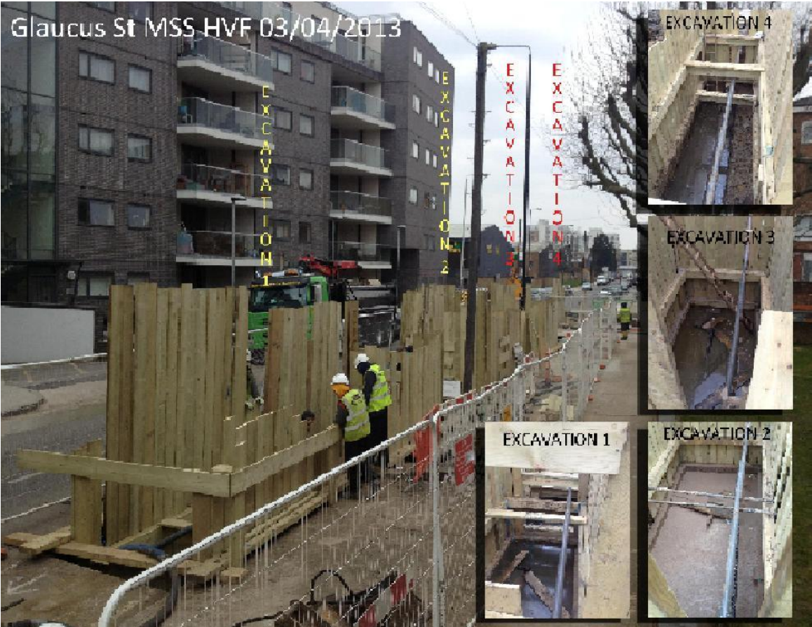
Figure 19: Composite views of the excavations and joint bays at Glaucus St.
