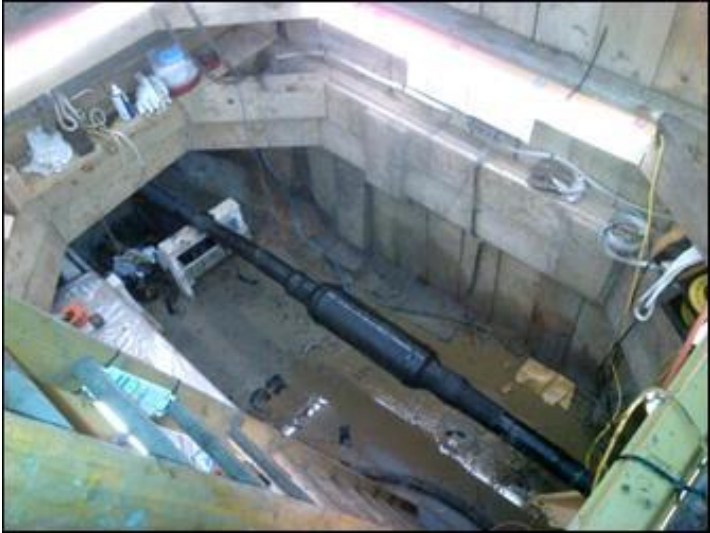
Figure 42: New Cable route circa 2m deep
