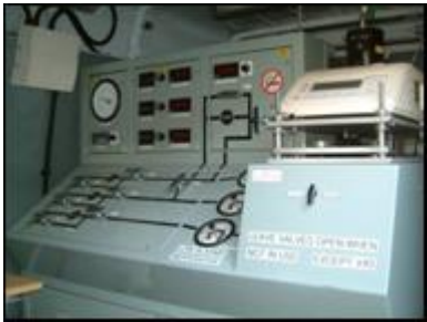
Figure 33: Vehicle mounted PFT Leak location equipment
