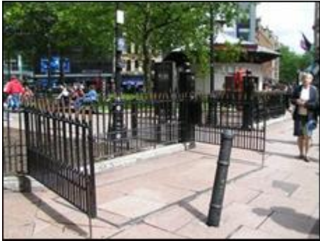
Figure 48: Personal access hatch at Leicester Square Substation
