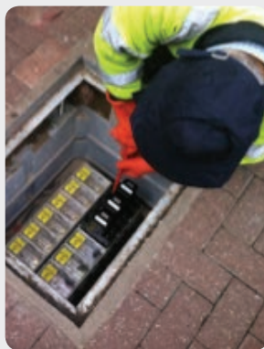
Retrofit switches being installed to a Link Box
