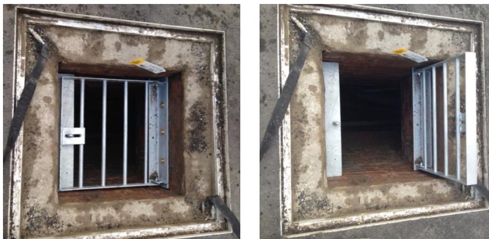
Figure 15: Example of fall arrest installation
