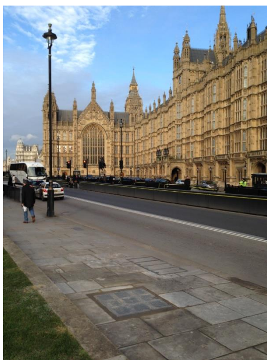
Figure 12: Example of FFP10 installation – Palace of Westminster
