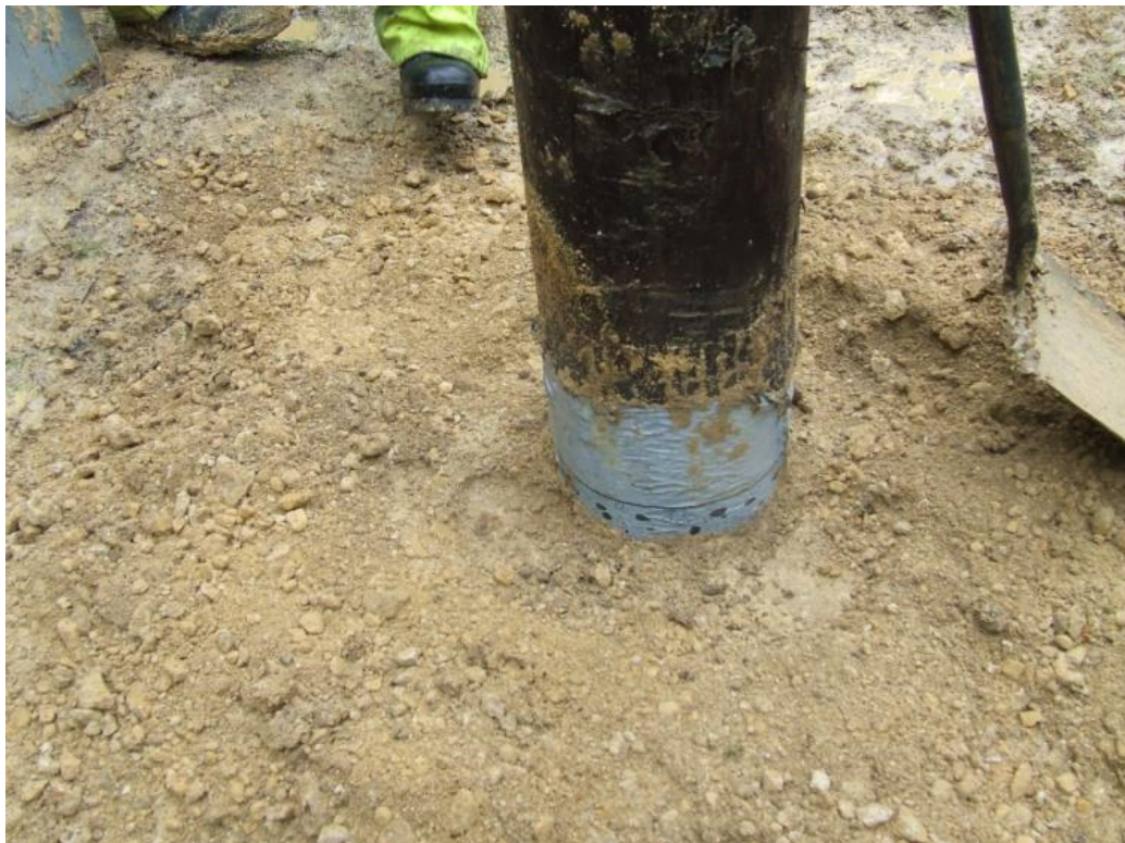
Figure 31 – Pole saver installed on a wood pole
