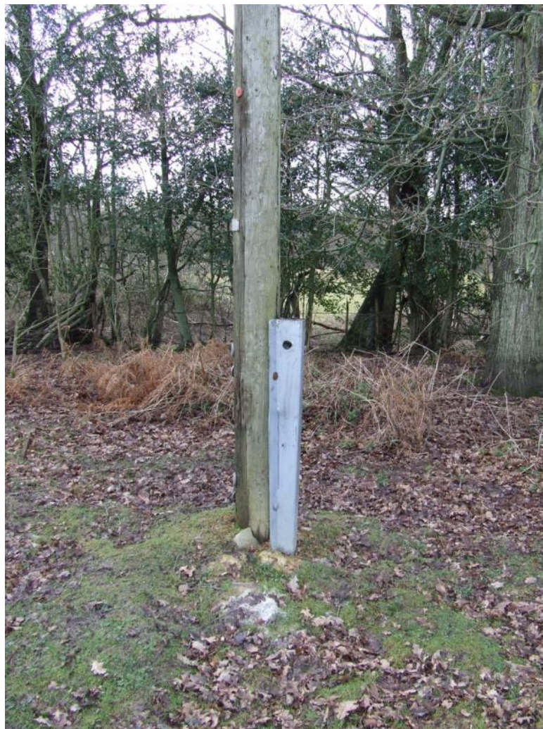
Figure 32 – Pole brace installed
