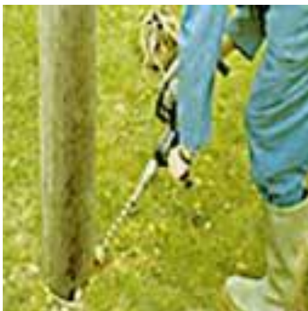
Figure 29 – Boron rod installation
