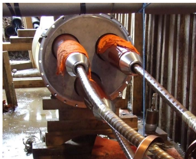
Figure 17 – Aluminium joint
