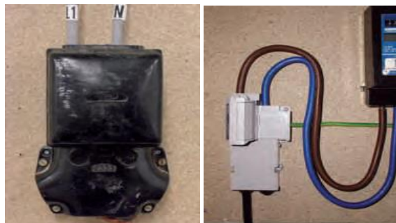
Figure 5 – Photos of Cut Outs
