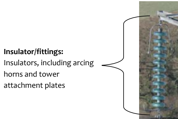
Figure 8 : Insulator/fitting (overhead tower line)
