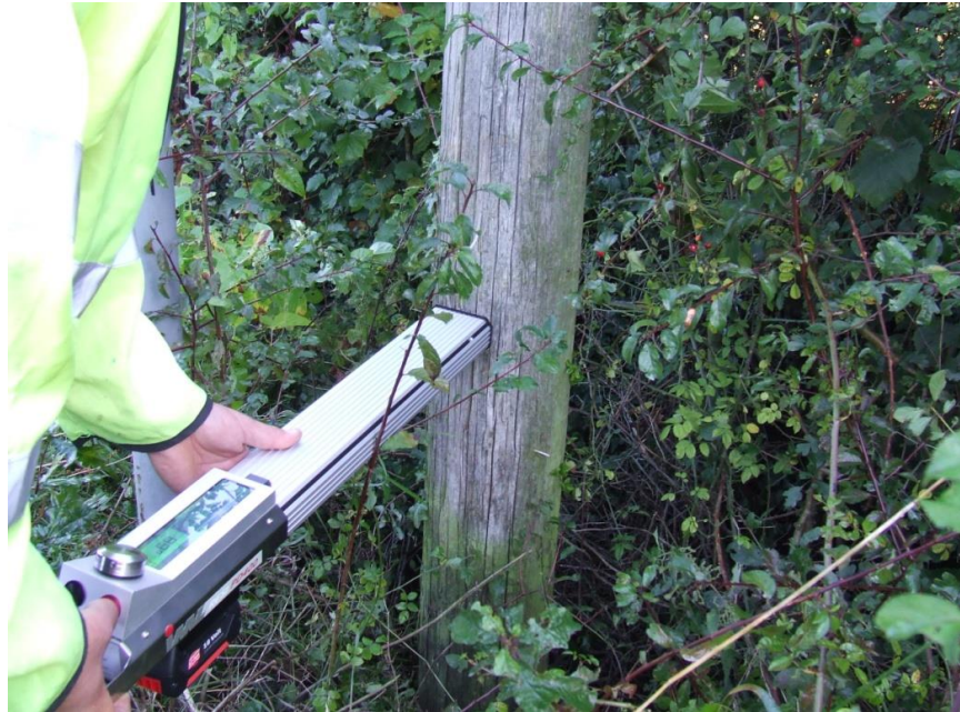
Figure 14 – Resistograph being used to determine extent of internal decay
