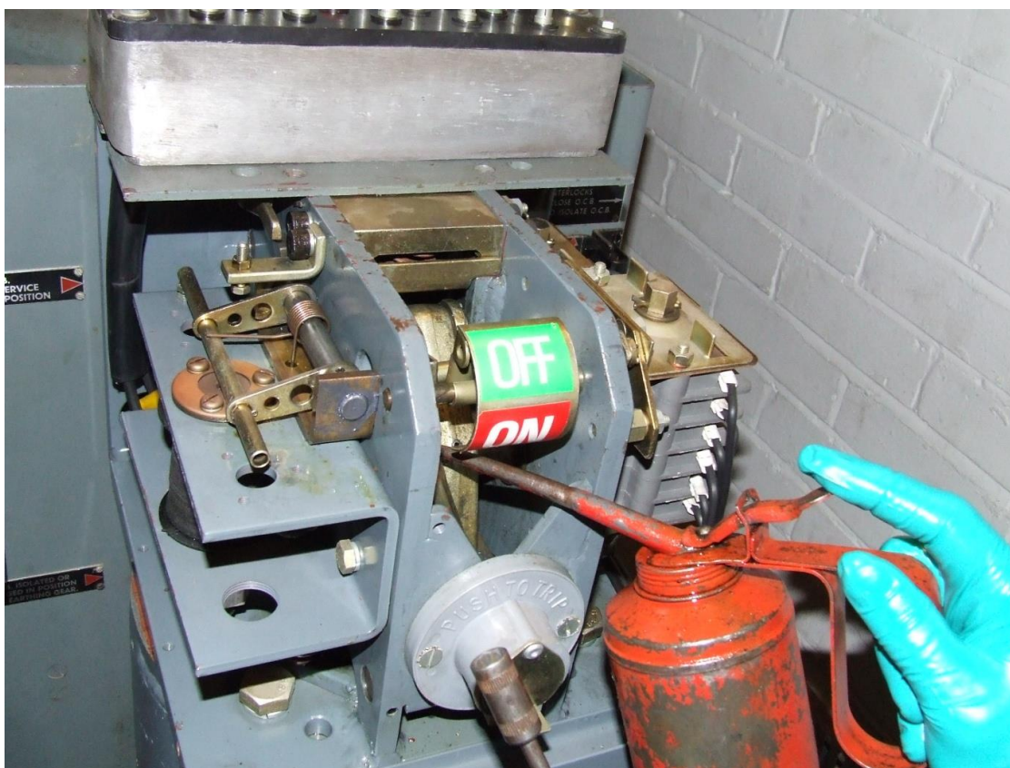
Figure 31– Carrying out mechanism maintenance on an oil circuit breaker
