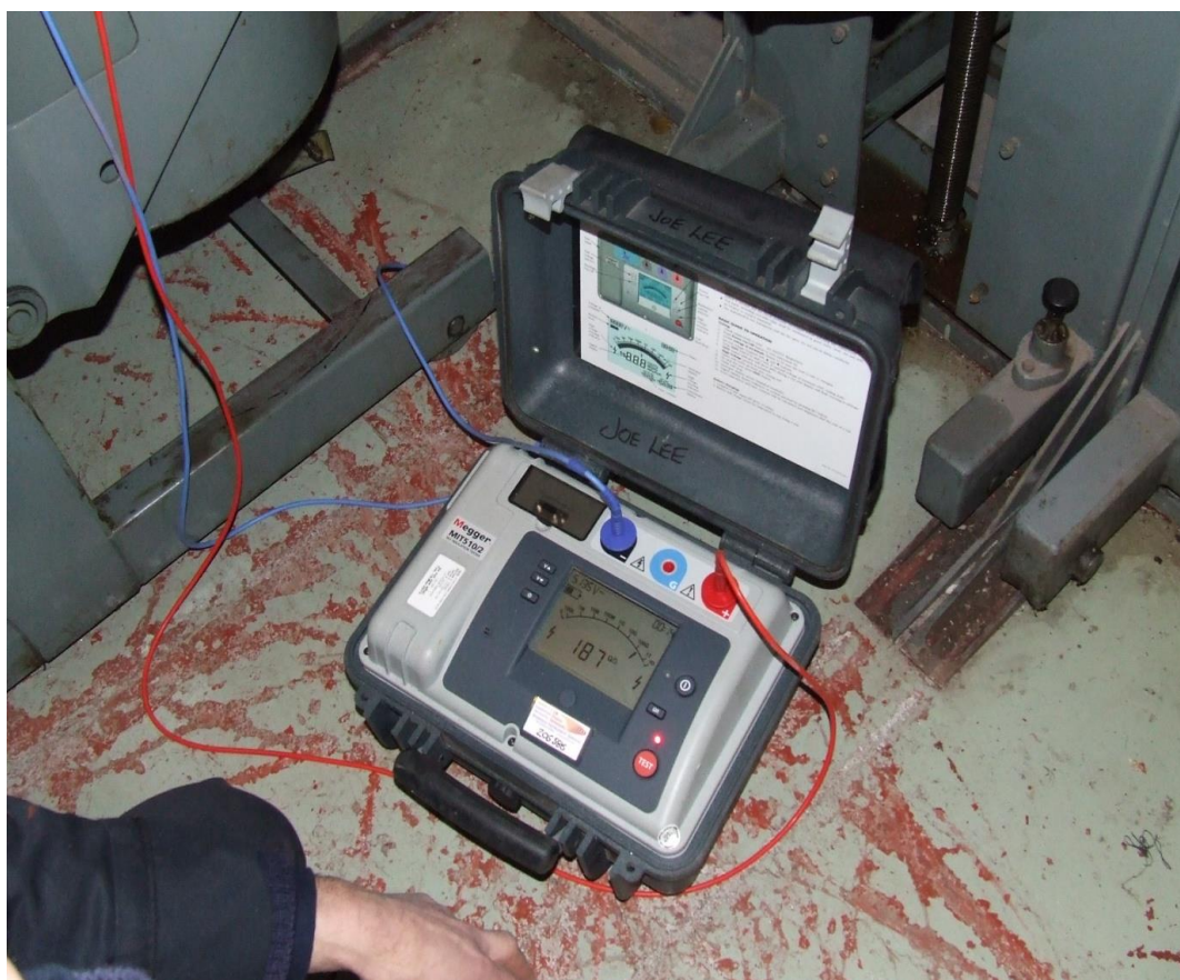
Figure 28 – Insulation testing of switchgear is important to understand its condition
