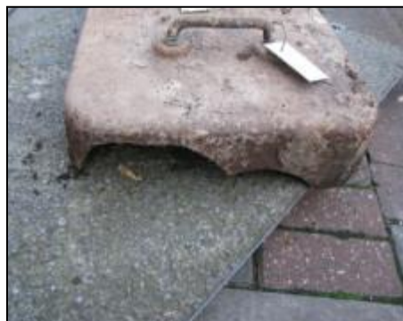
Figure 23: Broken Bell Cover
