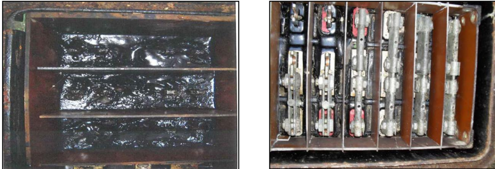
Figure 24: Example of High and Low Compound Level
