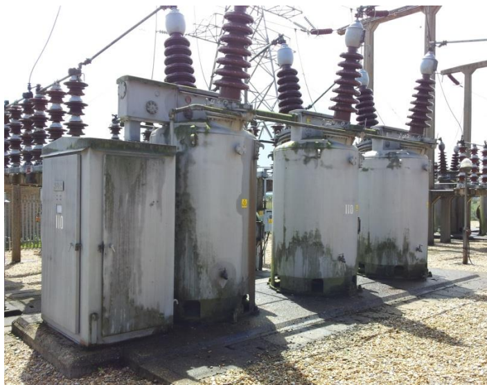
Figure 5 - GEC OFA11 Bulk Oil Circuit Breaker
