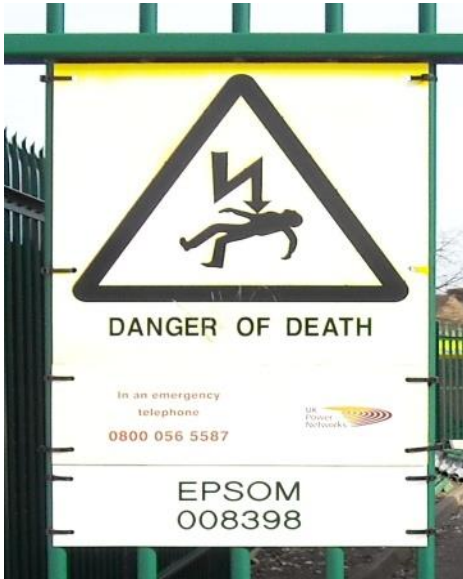
Figure 3 – Faded signage due to UV exposure
