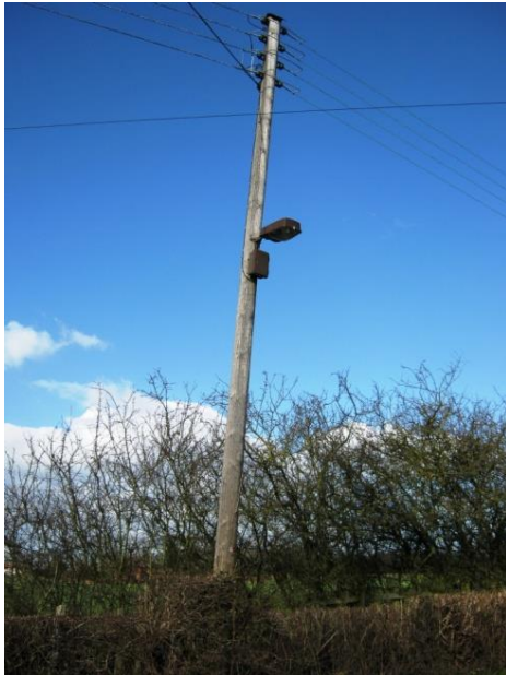
Figure 1– Signage missing/fallen off
