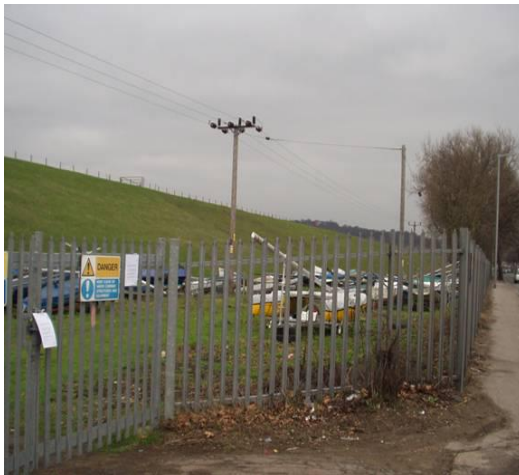
Figure 11- Boat storage yard; key-risk and high-risk mitigation
