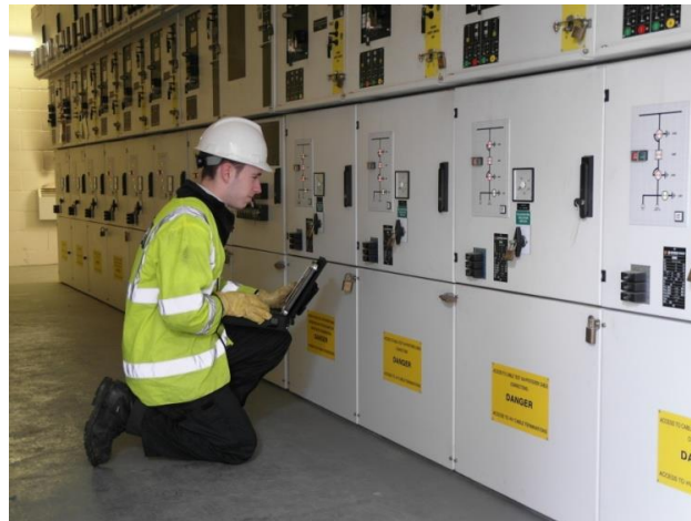
Figure 8 – Substation inspector with HHD
