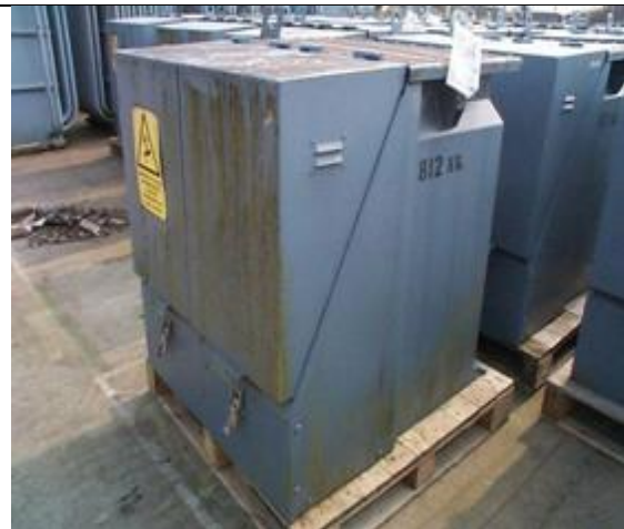
Figure 5: Replacement compact 2-3kV substation
