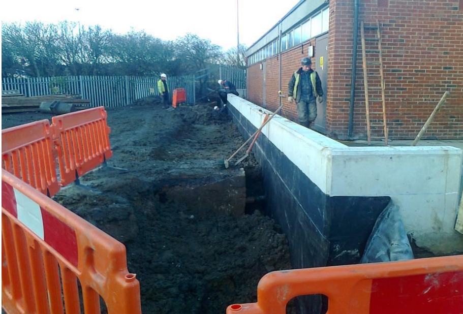
Figure 7 Flood defence works at Newhaven Grid
