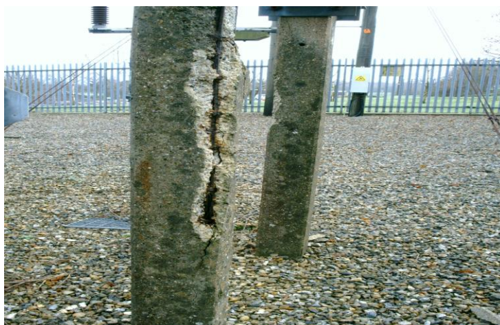
Steel cross primary – severe structural damage due for replacement in 2015-2016 as part of the substation major structure replacement programme (NAMP -1.47.64)
