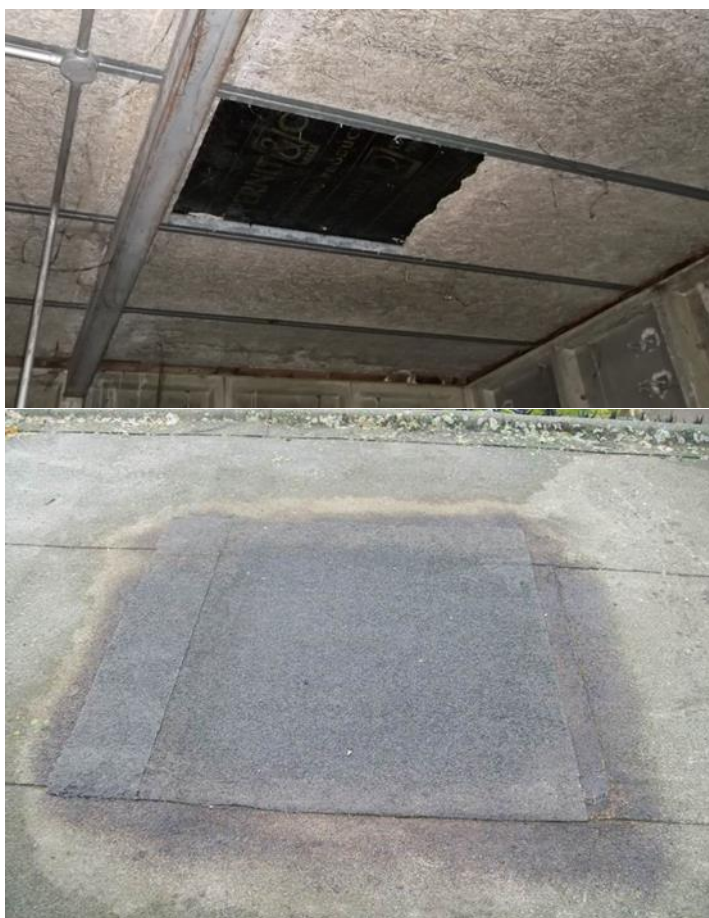
Typical Roof Repair
