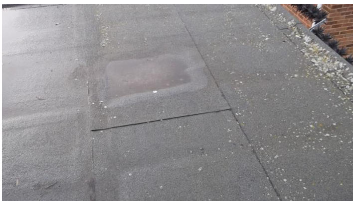
Figure 9b West Weybridge cable bridge (after mitigation works)
