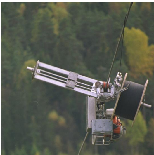
Figure 2 – The fibre wrapping machine at work
