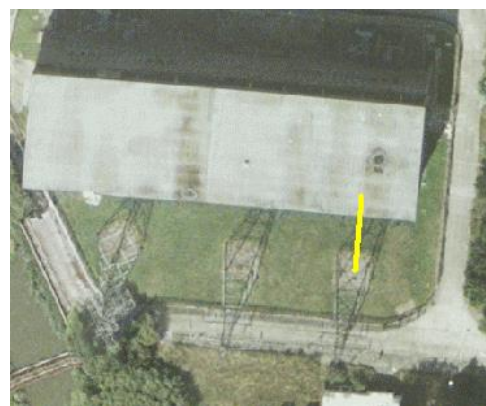
Terminal tower to relay room at Richborough
