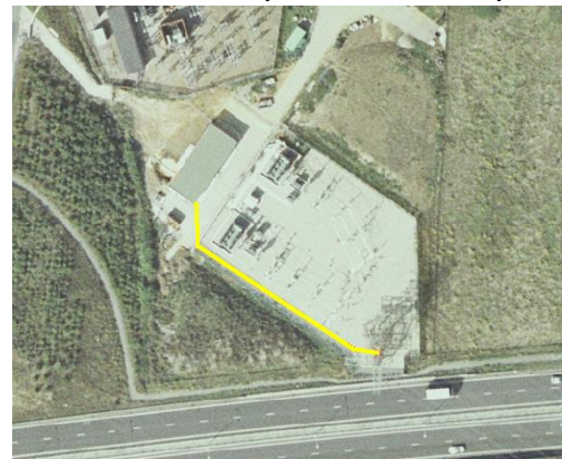
Terminal tower to relay room at Herne Bay
