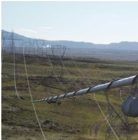
Figure 1 – Fibre wrap installed on an overhead line
