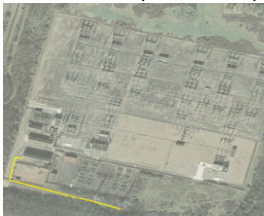
Terminal tower to relay room at Kemsley
