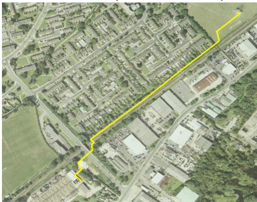
Terminal tower to relay room at Canterbury South
