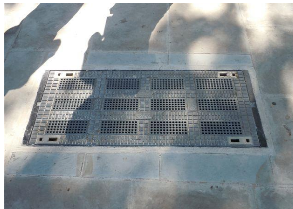
Figure 14: Structural Science Composites (SSC) 'S' Panel
