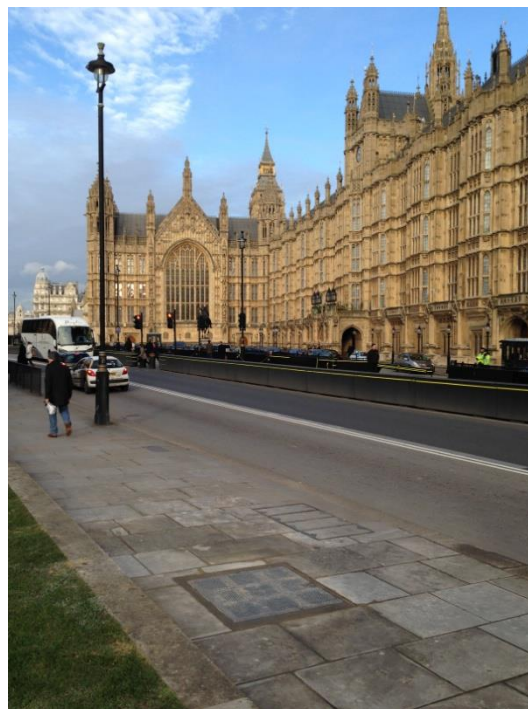
Figure 12: Example of FFP10 installation – Palace of Westminster
