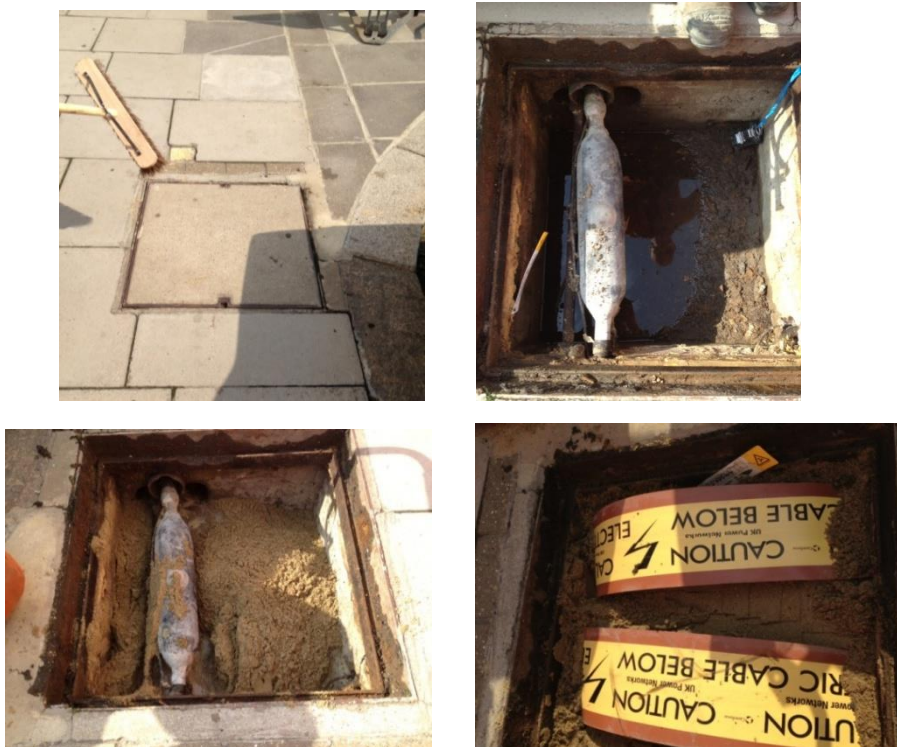
Figure 10: Example of Sand Infill Mitigations
