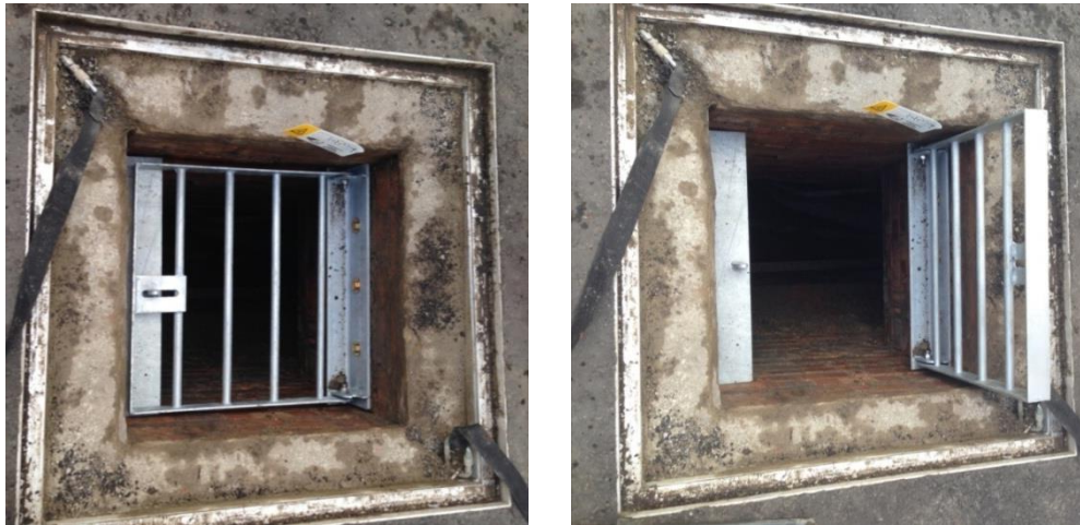
Figure 15: Example of fall arrest installation
