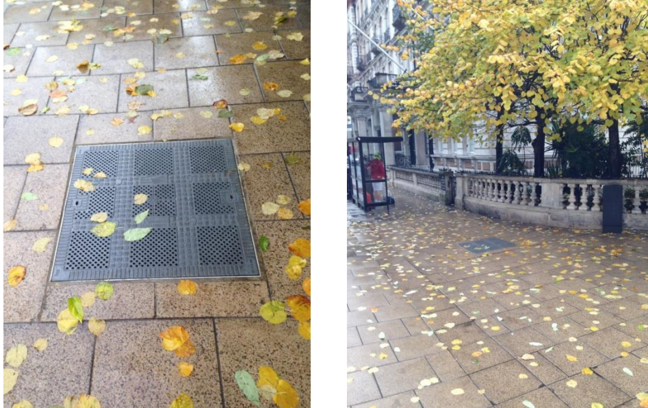
Figure 11: Example of FFP10 installation – Grosvenor Place
