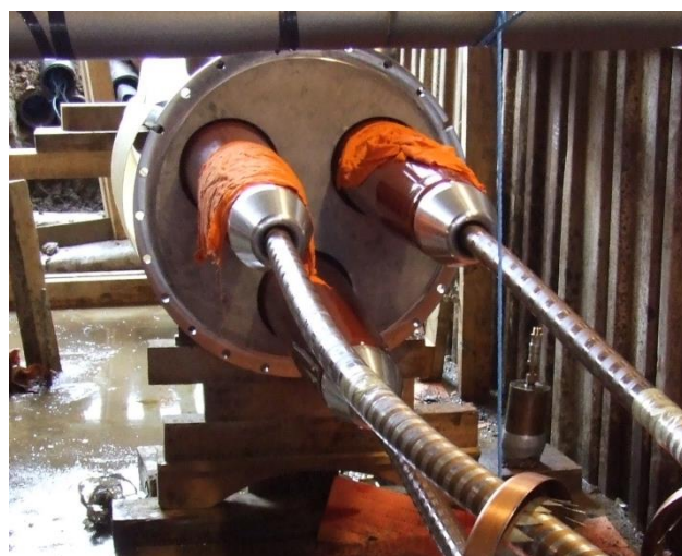
Figure 21 – Aluminium joint
