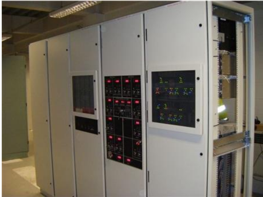
Figure 1 – RTU installation
