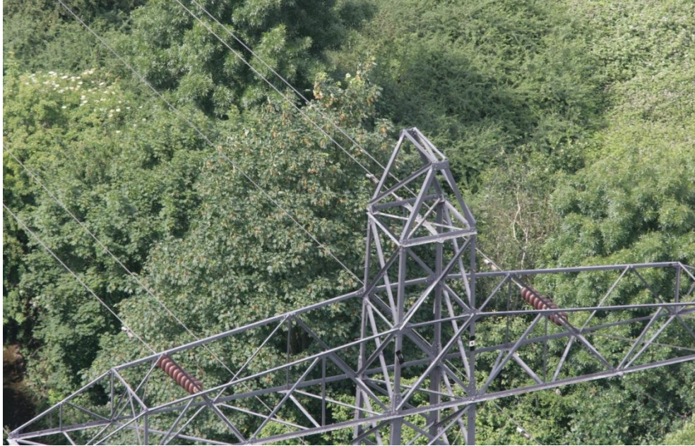
Figure 6: High-resolution image of a portion of an LPN tower
