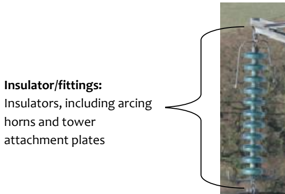
Figure 4 - Insulator/fitting (overhead tower line)
