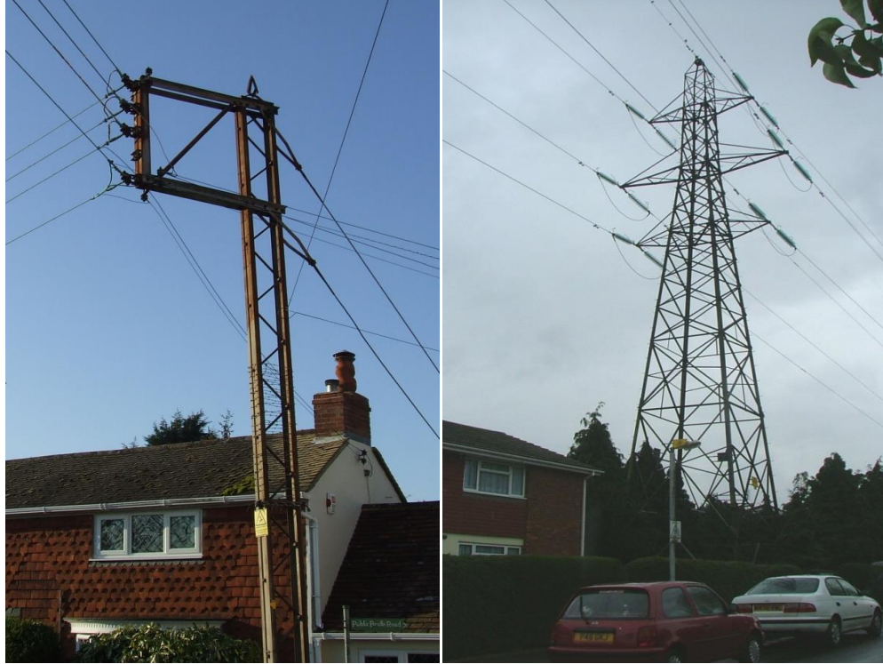
Figure 1: a narrow-based (left) and broad-based (right) tower, illustrating the differences in design and construction
