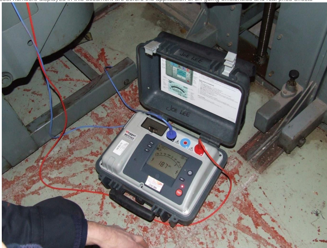
Figure 16- Insulation Testing of switchgear is important to understand its condition
