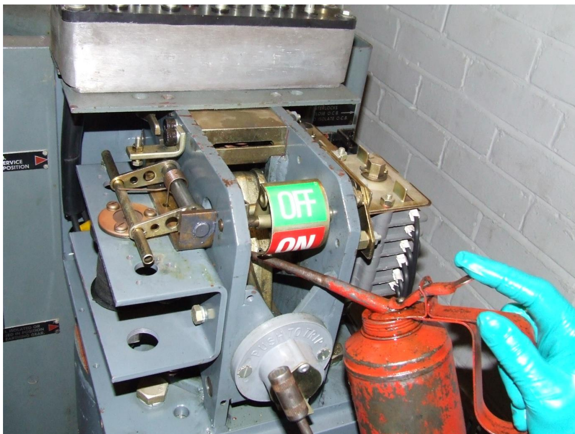
Figure 19– Carrying out mechanism maintenance on an oil circuit breaker
