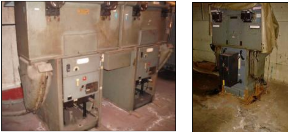
Figure 8: SCO RAE4 RMU at Queenhithe Hotel, Paternoster and SCO RA71 RMU
