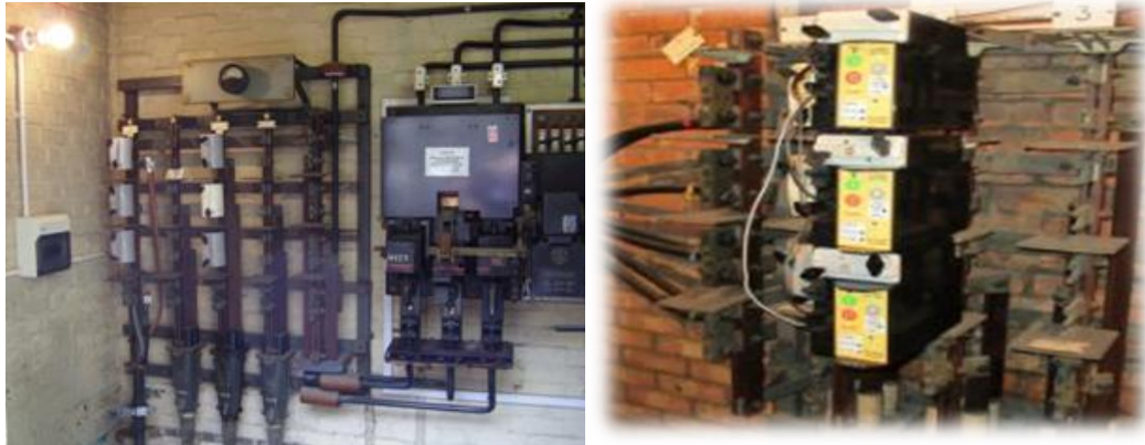
Figure 29: Before and After: LV CBs Installed on an LV Board
