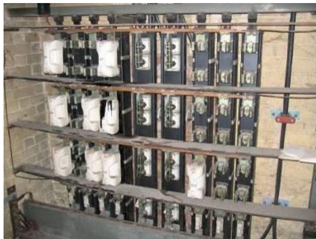
Figure 19: Non-Standard Fuse Carriers on Lucy LV Board
