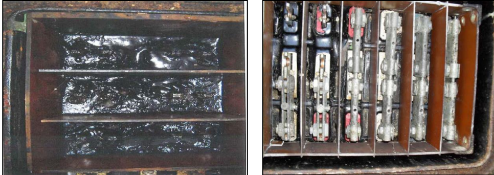
Figure 21: Example of High and Low Compound Level
