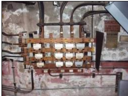
Figure 9: Westminster Board installed at Grosvenor Place 16 Substation
