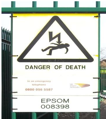
Figure 1 - Faded signage due to UV exposure
