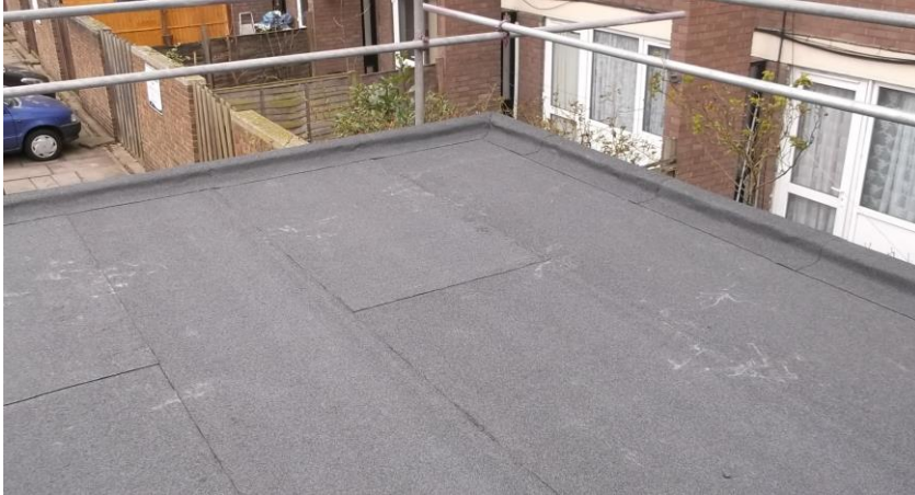
Figure 9 Replacement roof at Willington Road
