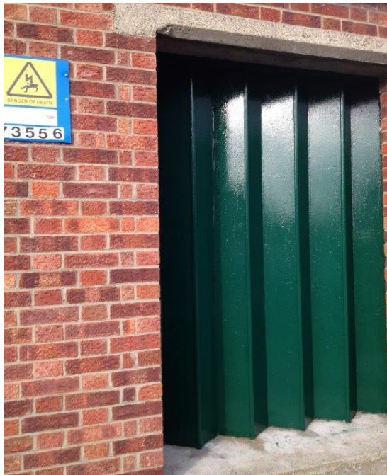
Figure 12 Door Refurbishment at Rossland Close
