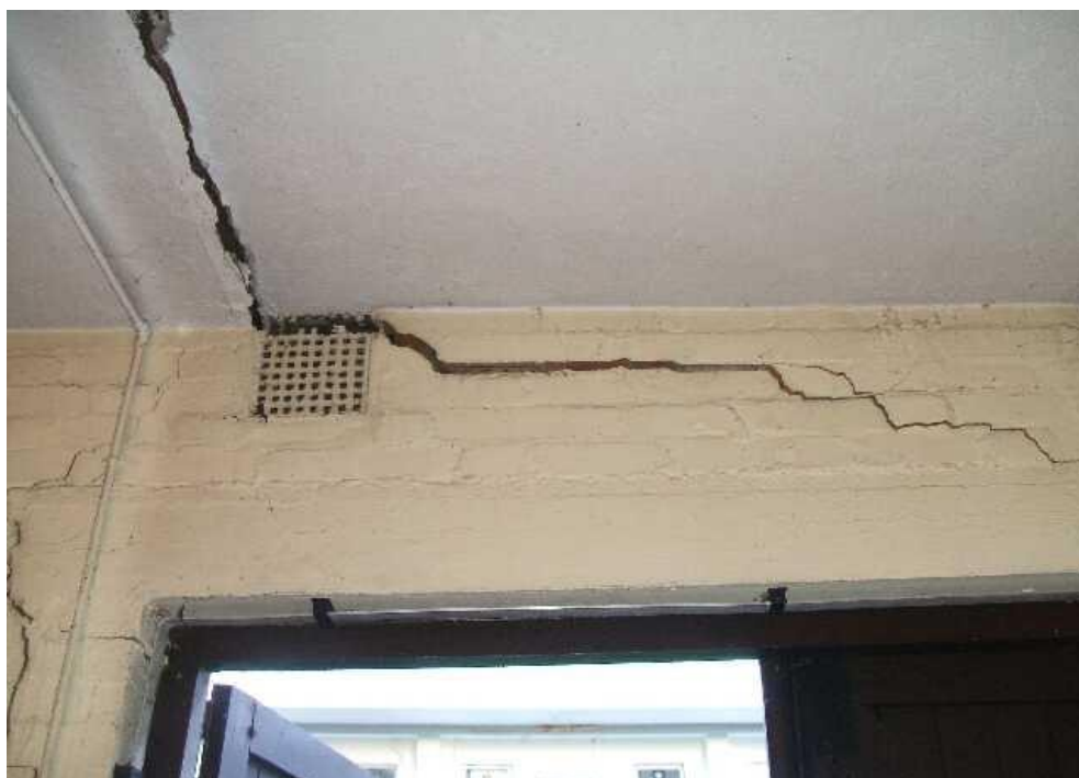
Bromley Grid 33kV – significant crack on building representing a Condition 4 building. Serious structural failure leads to more costly structural refurbishment expenditure.
