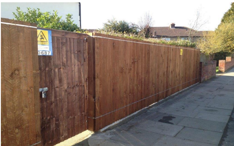
Figure 11 Surround Replacement at Rochester Avenue
