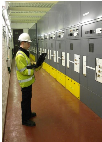
Figure 8 – Substation inspector with a handheld device
