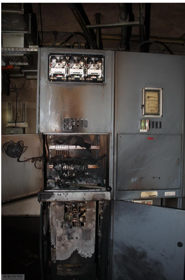
Figure 18 – GEC VMX: Failed 11kV panel
