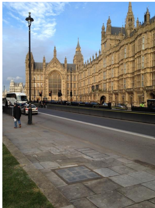
Figure 12: Example of FFP10 installation – Palace of Westminster
