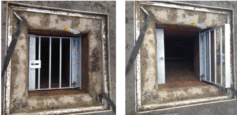
Figure 15: Example of fall arrest installation
