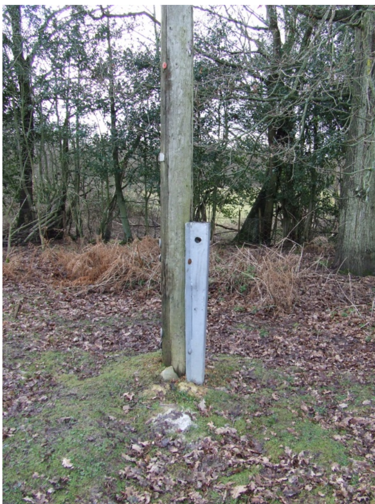
Figure 33 – Pole brace installed
