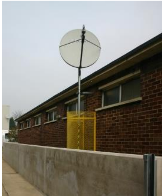
Figure 2 – Substation VSAT
