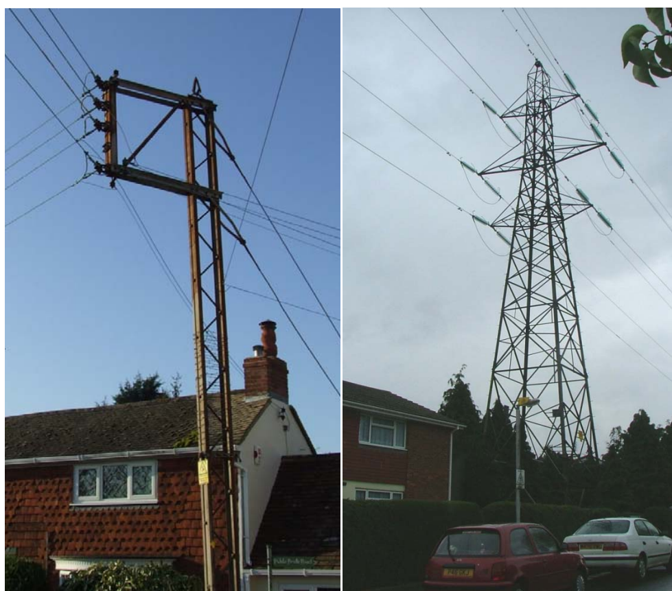
Figure 1: A narrow-based (left) and broad-based (right) tower, illustrating the difference in design and construction
