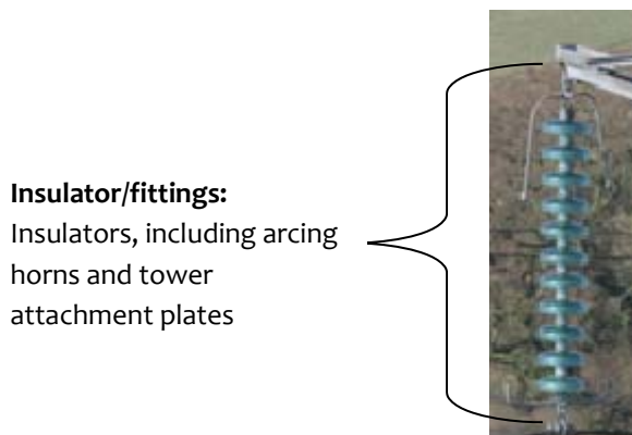
Figure 8 : Insulator/fitting (overhead tower line)
