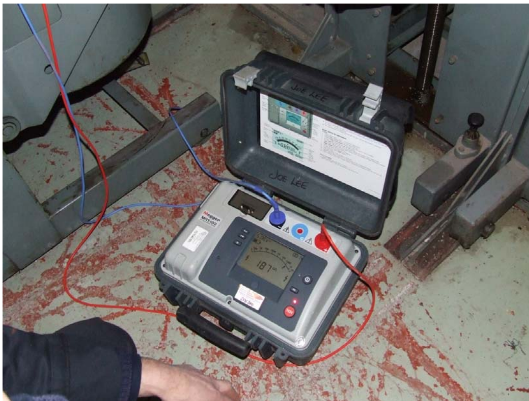
Figure 27 - Insulation testing of switchgear is important to understand its condition
