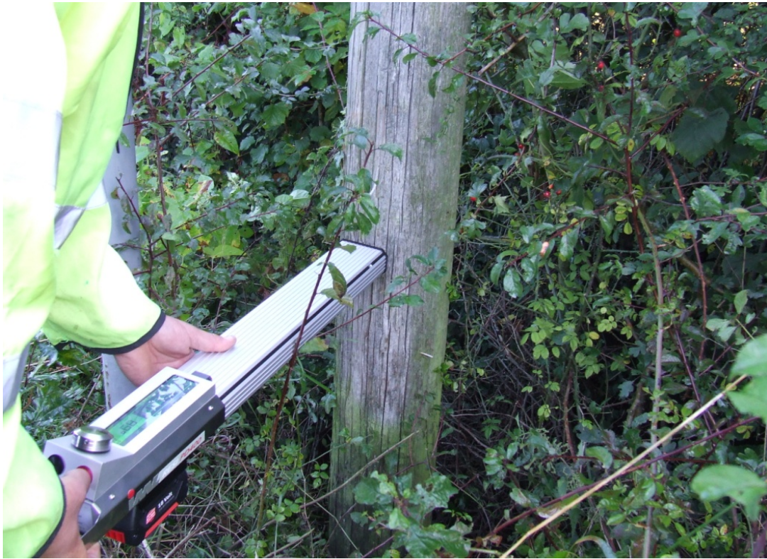
Figure 13 - Resistograph being used to determine the extent of internal decay
