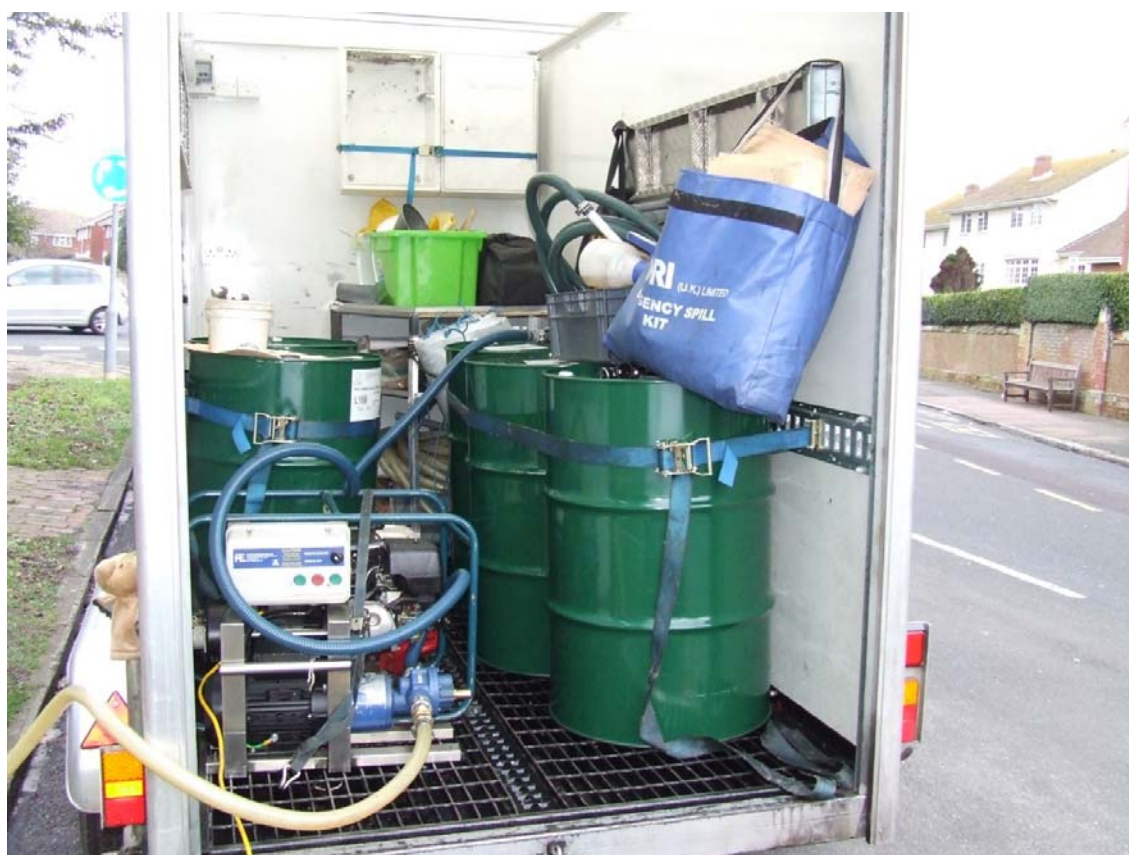
Figure 35 - Secondary substation maintenance oil handling facilities
