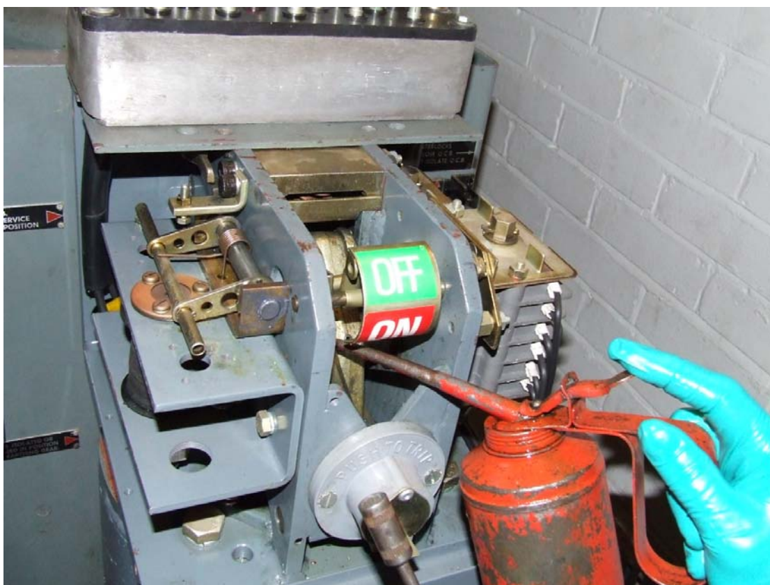
Figure 28 - Carrying out mechanism maintenance on an oil circuit breaker
