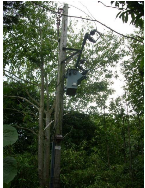
Figure 12 – Climbable tree issue; priority varies from P3 to P5 depending on the ESQCR risk rating
