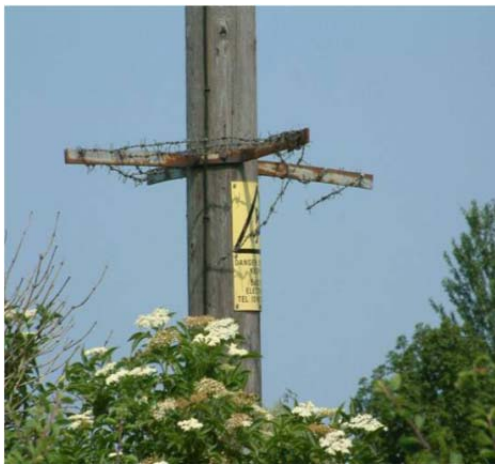
Figure 7 – Defective anti-climbing device; priority is P3 or P4 depending on the ESQCR risk rating
