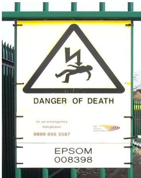
Figure 3 – Faded signage due to UV exposure
