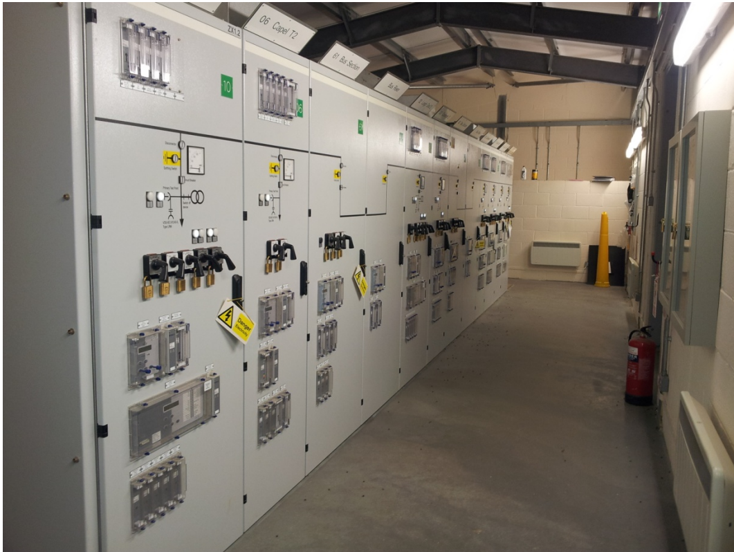
Figure 10 – ABB ZX1.2 switchboard
