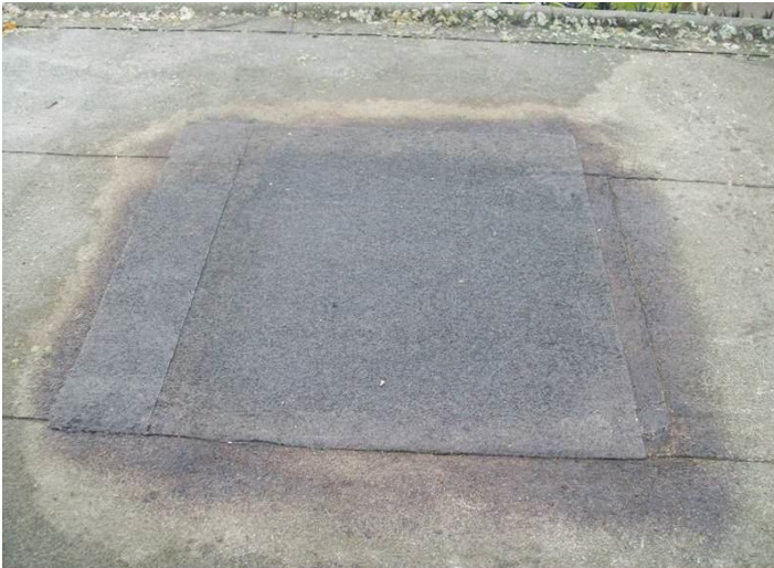
Typical Roof repair
