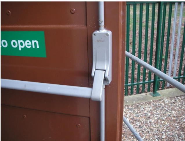
Door handle replacement
