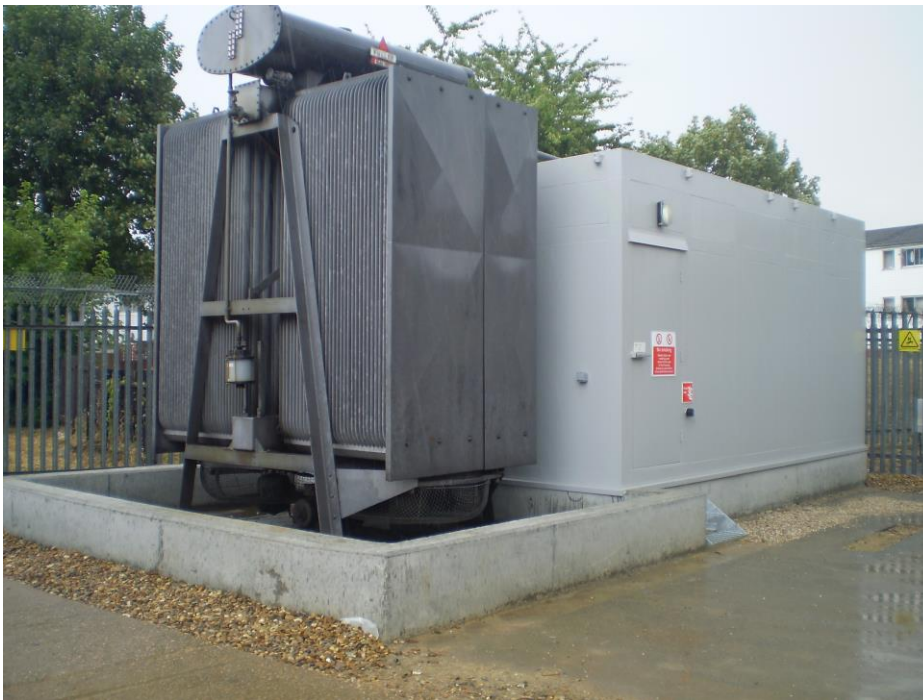
Figure 10 Central Tottenham- completed transformer oil bund
