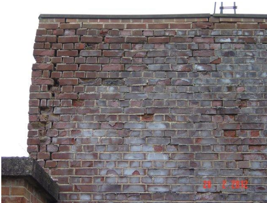
Figure 7 Epping Grid transformer housing representing a Condition 4 building.
