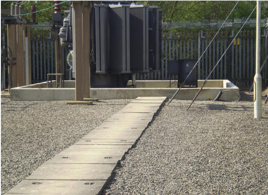
Figure 11 Farcet primary – completed transformer oil bund
