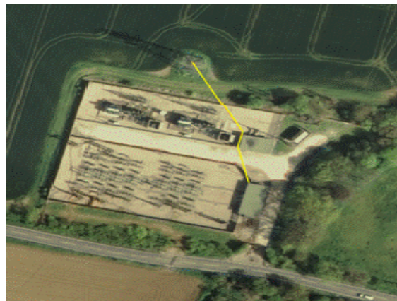
Terminal tower to relay room at Fleethall
