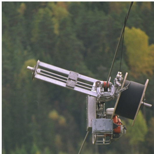
Figure 2 – The fibre wrapping machine at work
