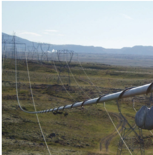
Figure 1 – Fibre wrap installed on an overhead line
