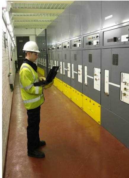
Substation inspector with a handheld device
