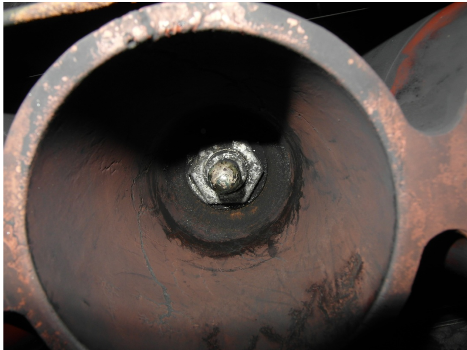
Figure 20 – GEC VMX: Tracking inside circuit spout
